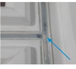
»\*If there is an intersecting mull, first fill cavity full of silicone, then down each side of the mull channel. Also, fill accessory grove about 1"in each direction. Finally, tool/smooth silicone in all directions.
