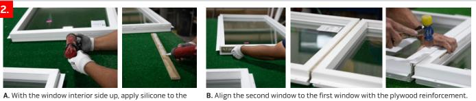
**First frame without the nail fin.** Next, place the plywood
