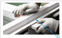
»-Then fill the rest of the cavity the same way all the way down to the bottom side of the plywood reinforcement.
