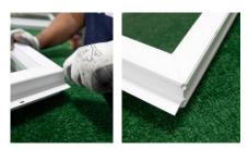
C. Where the nail fin was removed, square up the corners by removing excess vinyl weld from each corner. Do this for each end, interior and exterior of the window.
