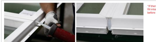
\*If there is an intersecting mull, fill intersection with silicone before applying cover
